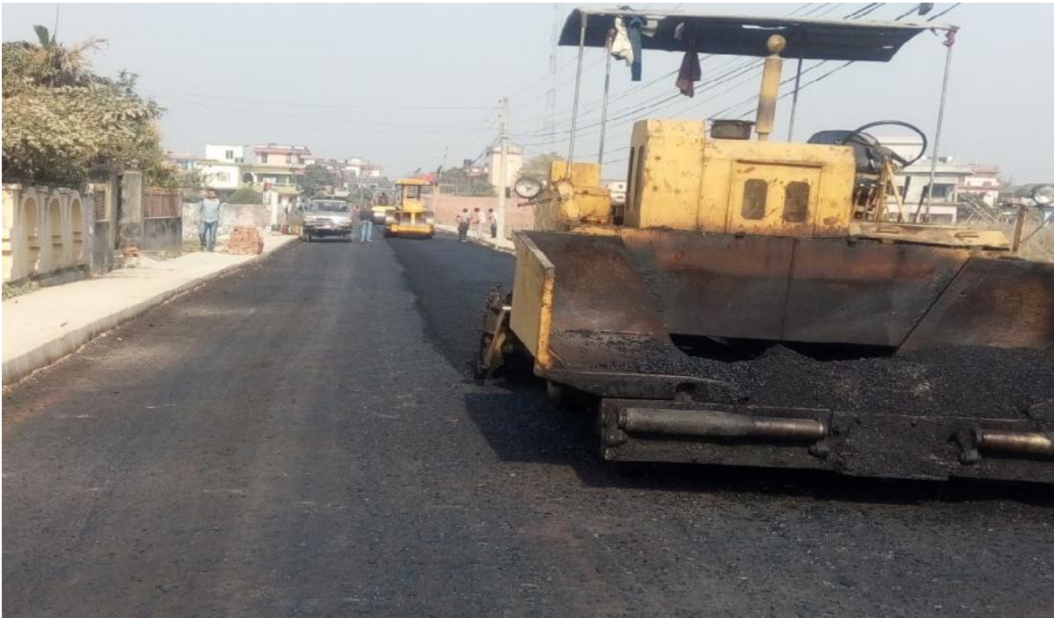
Laying and compaction of Asphalt concrete work at Kailash path, Siddharthanagar
