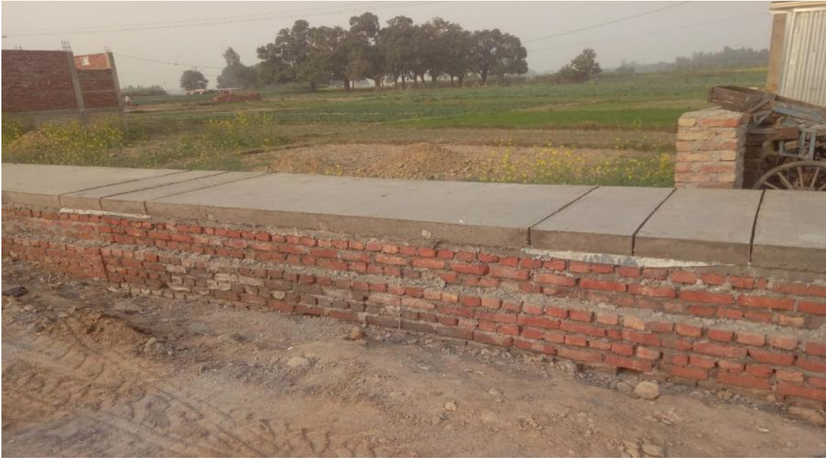
Drain Covered Slab, Ganesh man Chowk, Siddharthanagar
