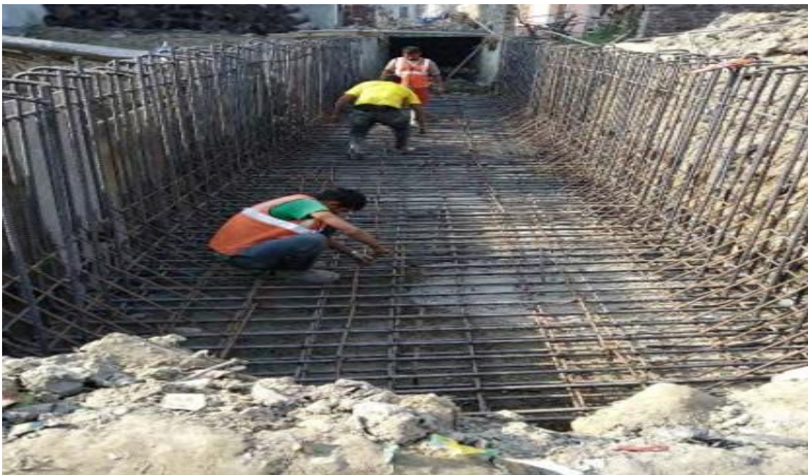
Re-bar erection work for Changbari Nala, Biratnagar
