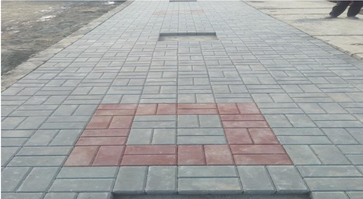
Footpath construction at Bimanghat road, Nepalgunj
