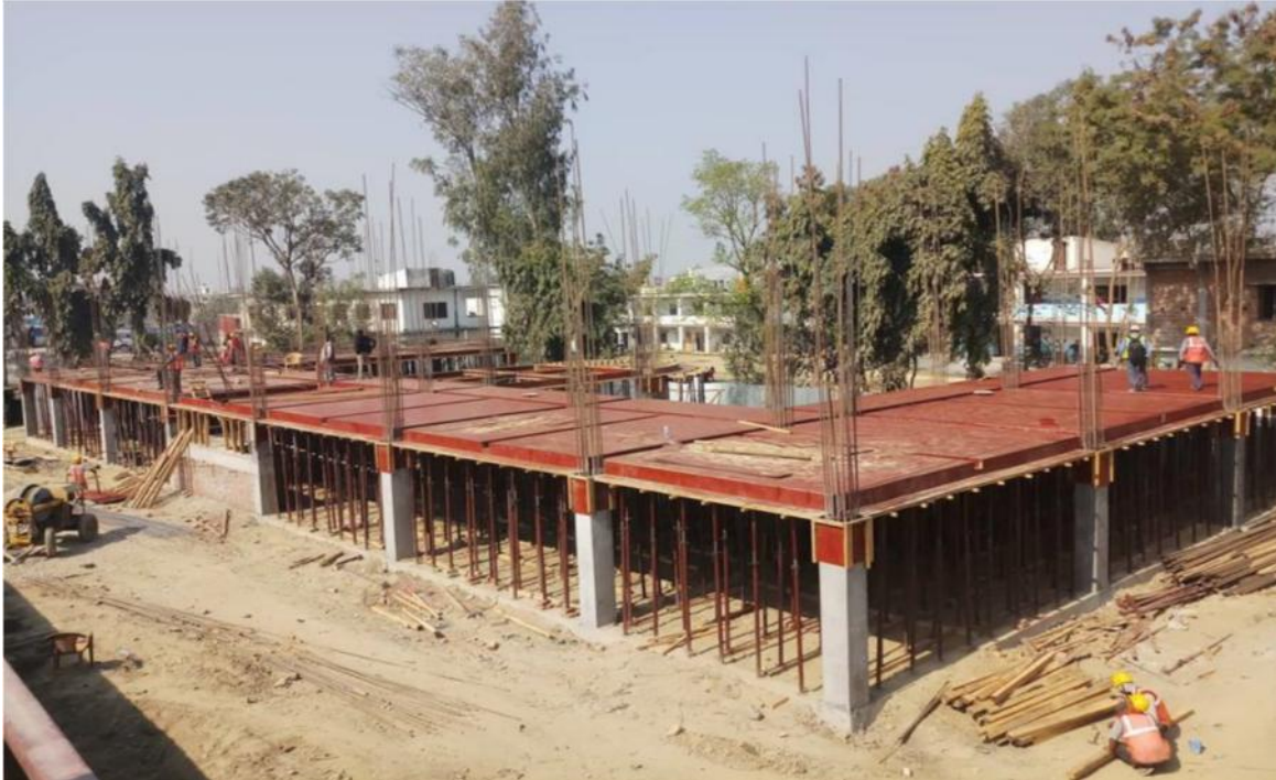
Construction of School Building on progress, Birgunj
