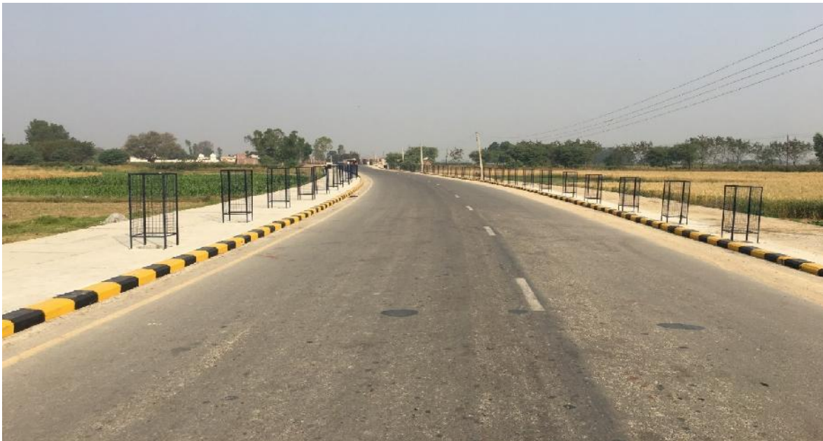
Completed Road Section at Ganeshman Singh Chowk to Paraspur Road, Nepalgunj
