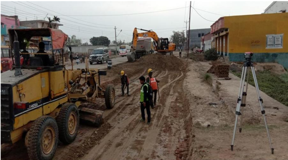
1 st By-Pass, Preparation of Sub Grade and Sub-Base Work, Birgunj
