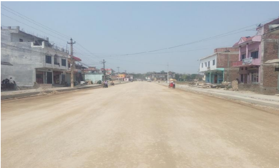
Base course laying of stadium road, Siddharthanagar
