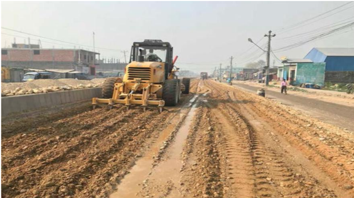
1st By-Pass Road, Sub-base grading Work, Birgunj
