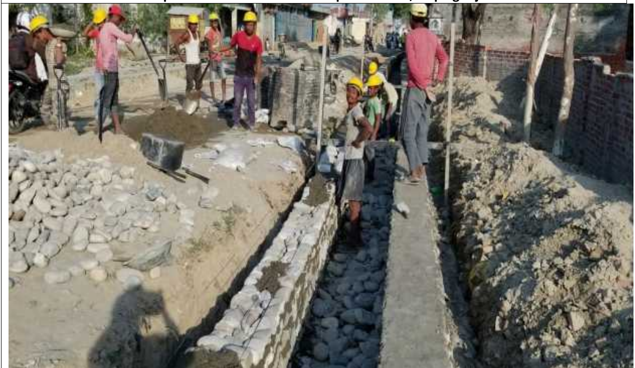
Stone Masonry Drainage work, Nepalgunj
