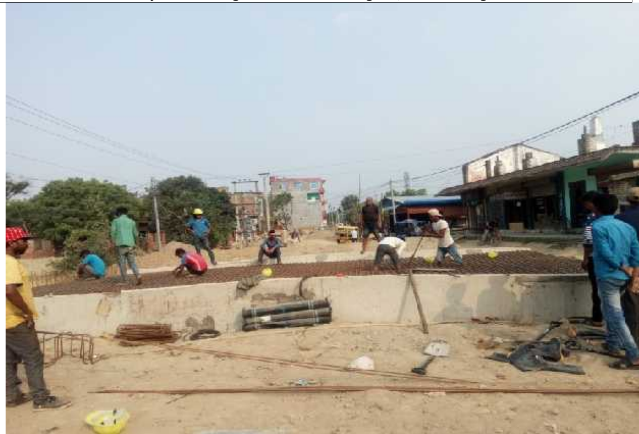
Slab Reinforcement at Danda Khola, Siddharthanagar
