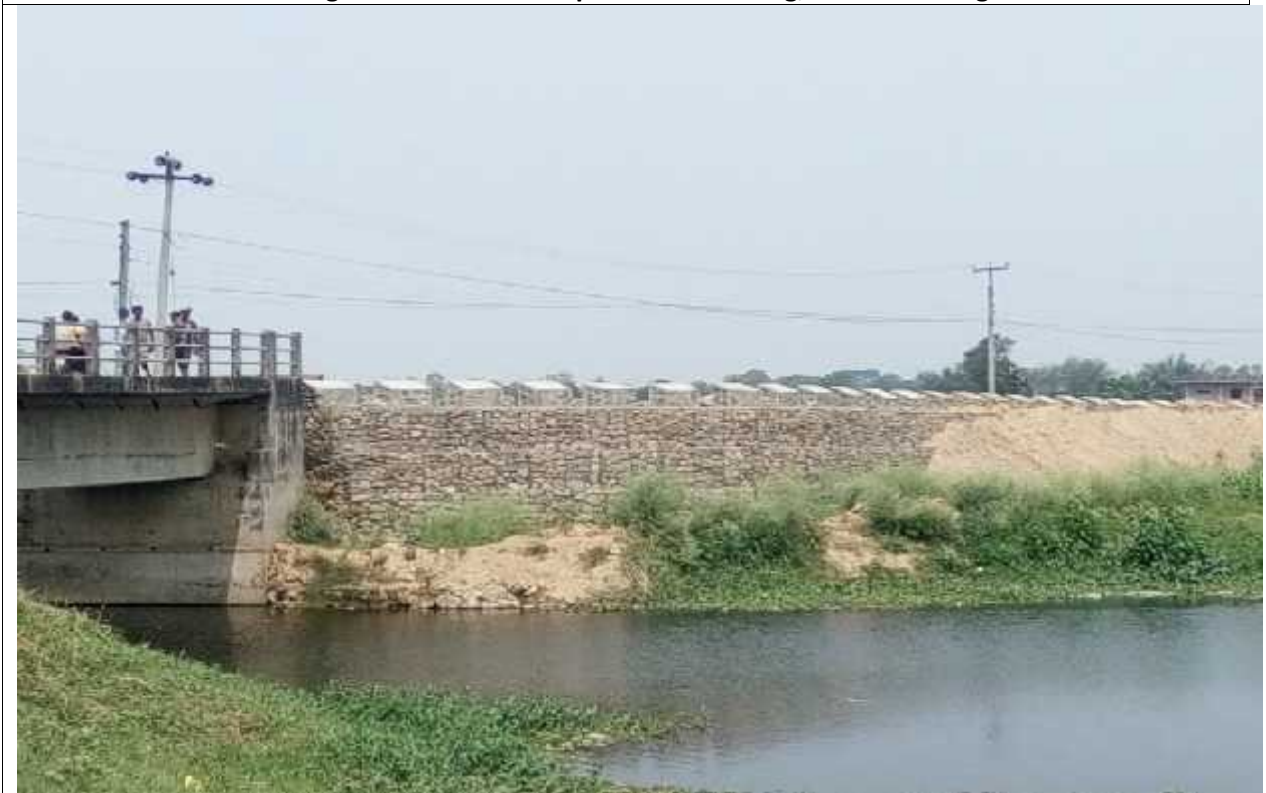
Gabion Retaining wall for Sima Path, Siddharthanagar
