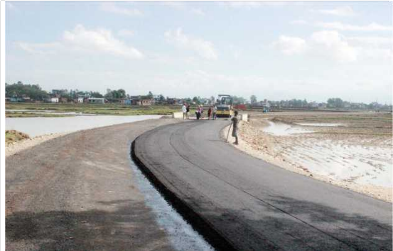
Asphalt concrete work at Pilaripurwa Road, Nepalgunj
