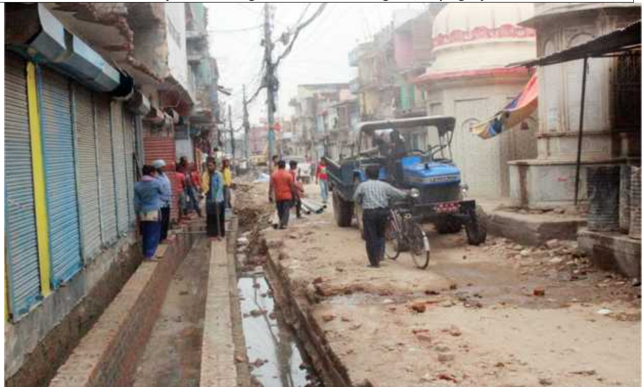
Drainage Construction work, Nagarbhawan to Tribeni chowk, Nepalgunj
