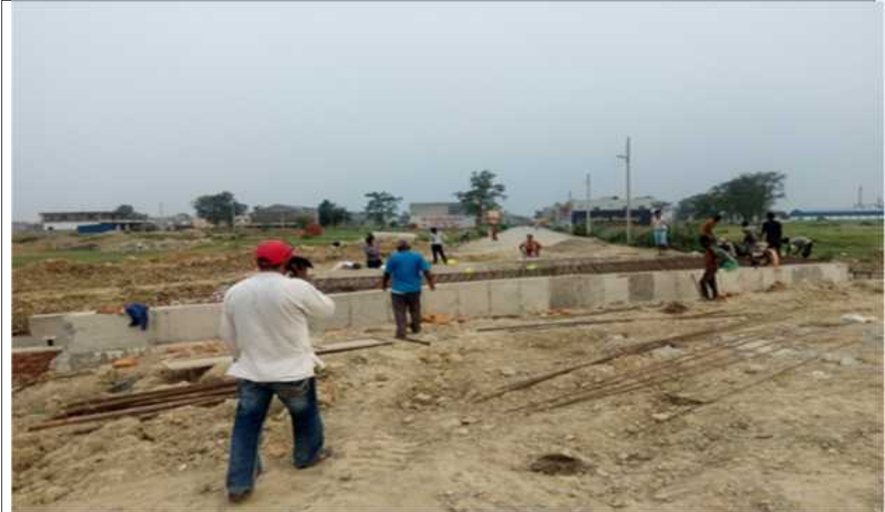
Working Slab Culvert for Airport Nala Crossing, Siddharthanagar
