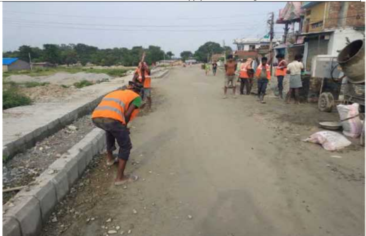
Laying of kerbstone's, Biratnagar
