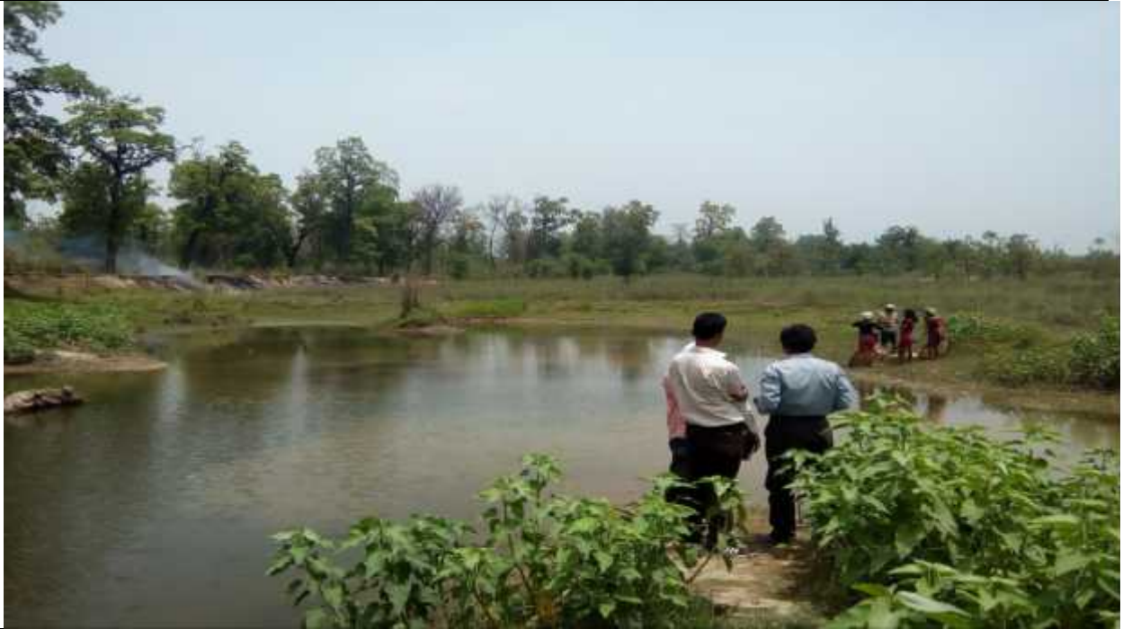
Ponding of water in proposed ISWM Facility of Godavari Municipality
