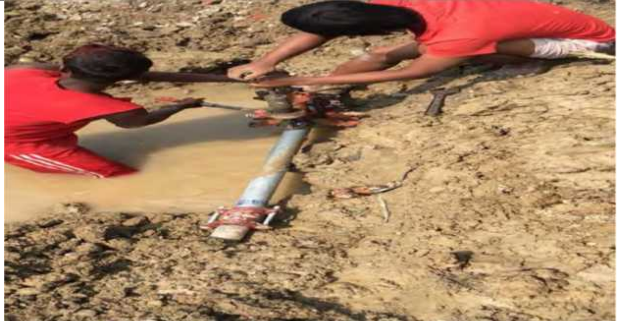
Reinstatement of water supply work, Biratnagar
