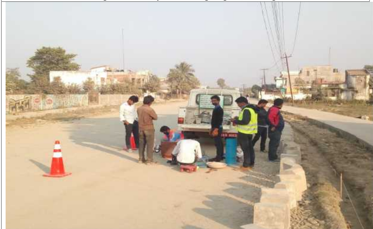
Base course on site compaction test, Biratnagar
