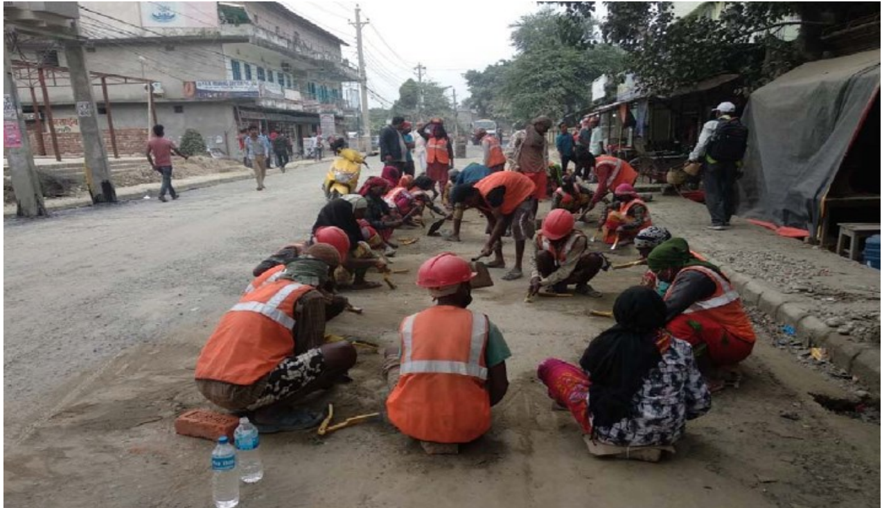
Brooming work at R41, Jahada Marga, Biratnagar
